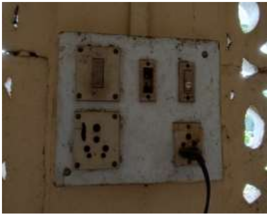
Save Energy Message Should be Displayed on Each Board
